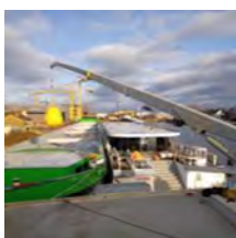
Hoisting, piling & lifting
